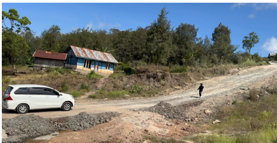
Figure 3. Poor infrastructure conditions in the Tourism Area of Fatumnasi Source: Primary data, 2024
